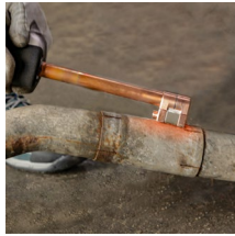
Removing exhaust pipes
